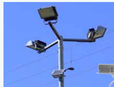
Repeater with optional Solar Panel for fully autonomous operation
